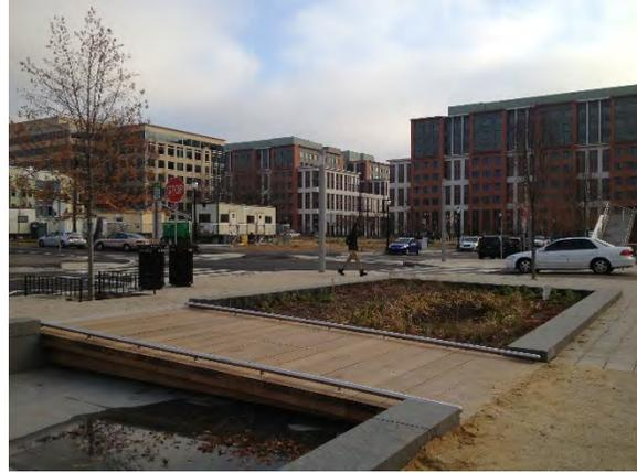
*Examples of how bioretention facilities can be incorporated into plaza designs.*
