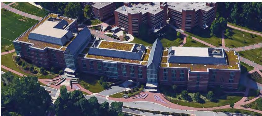
*The College of Liberal Arts Building has a green roof which helps with storm water management, extends roof life, and assists in insulating the building.*
